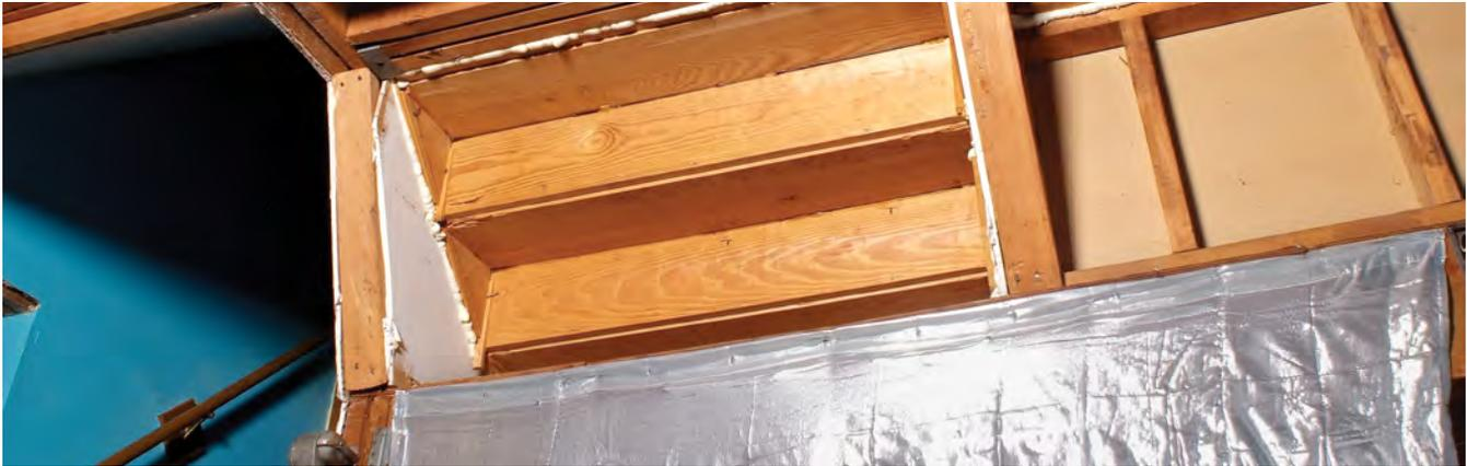
CRITICAL GAPS IN THE BASEMENT AND ATTIC WERE ADDRESSED WITH THE APPLICATION OF FOAM INSULATION.
