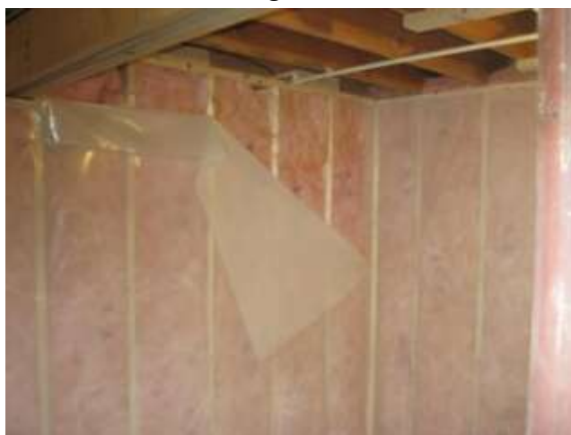
Figure B-2: Grade II Fiberglass Batts—Basement Walls
