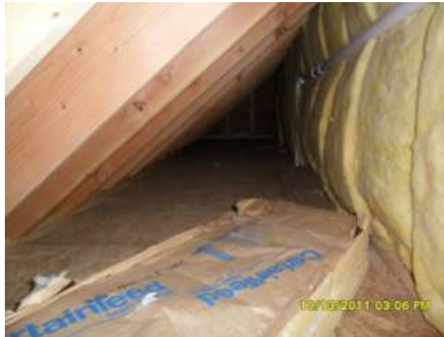
Figure B-3: Grade III Fiberglass Batts—Attic Kneewalls
