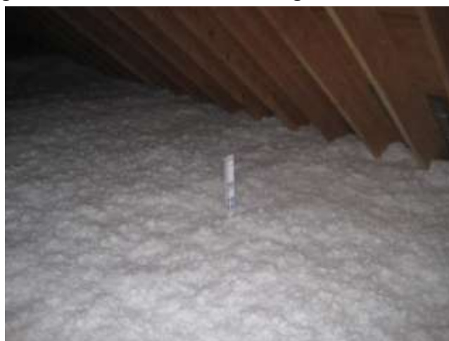
Figure B-6: Grade I Blown Fiberglass—Attic
