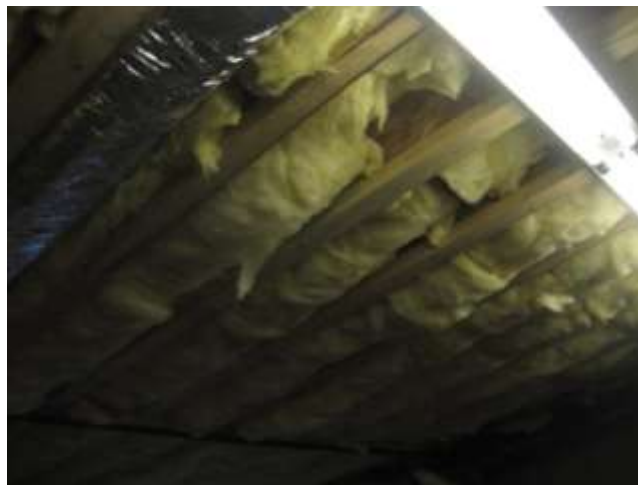
Figure B-5: Grade III Fiberglass Batts—Frame Floor
