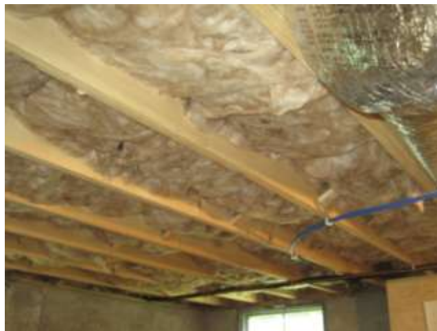
Figure B-4: Grade II Fiberglass Batts—Frame Floor
